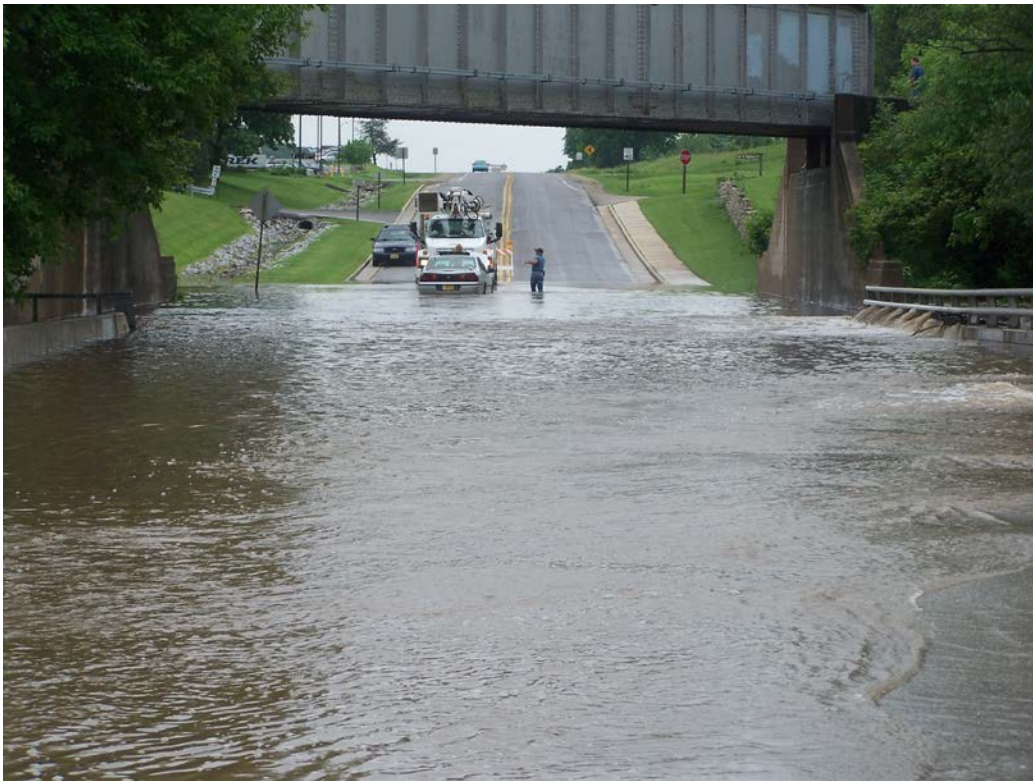
Figure 3. Flood Scenes from June 2008 in the City of Waterloo
